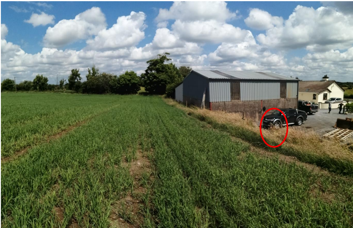
Appendix Figure B-3. Location C Installation
